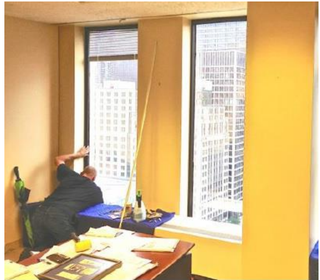
Thermolite's interior window system being installed on west-facing offices.
